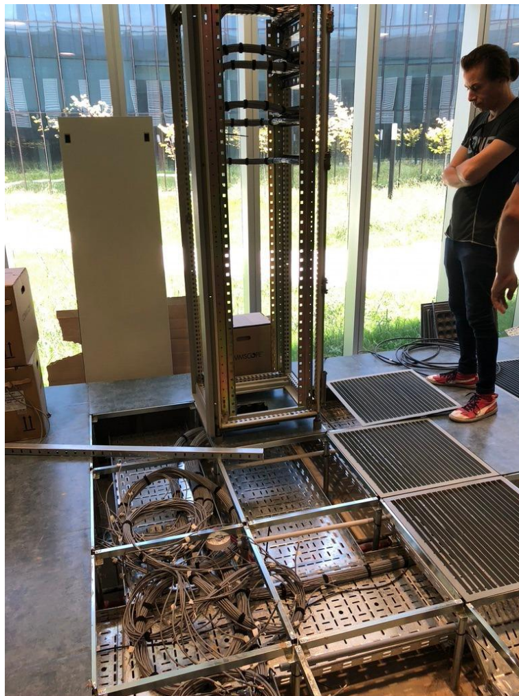
Figure 2: New computer center under construction, future home of our new server.
